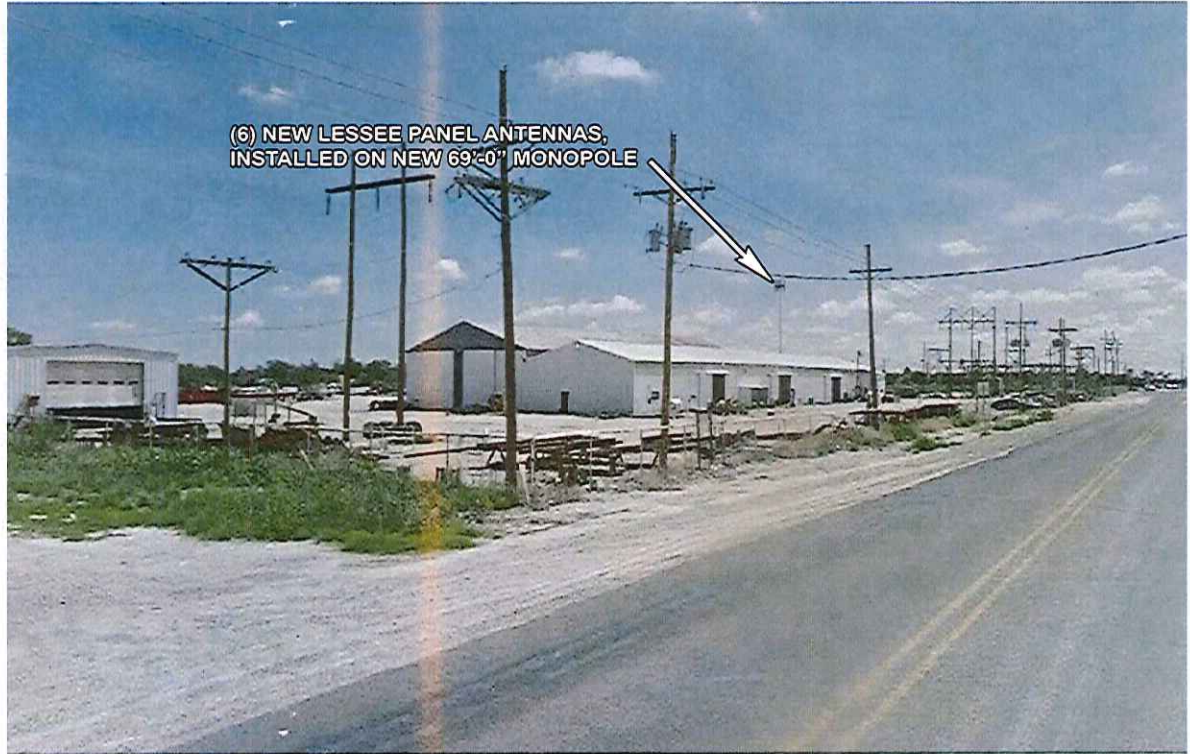
SOUTHWEST ELEVATION (LOOKING NORTHEAST)
